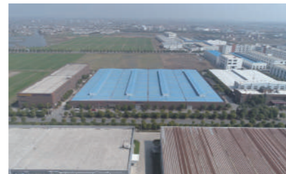
Xiangcheng production base In May 2012, Xiangcheng COZY company went into operation, it designed and produced HOUSETEC type for top five Japanese bathroom manufacturer.
