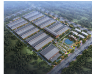
Hebei Hengshui production base Our factory area is 200,000m 2 , the annual Prefab Bathroom Unit production capacity is 250 thousand sets.
